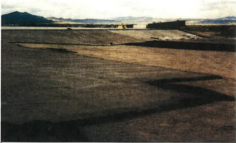
Photo 3. Concrete fill in geocells performs similar to concrete channels.
