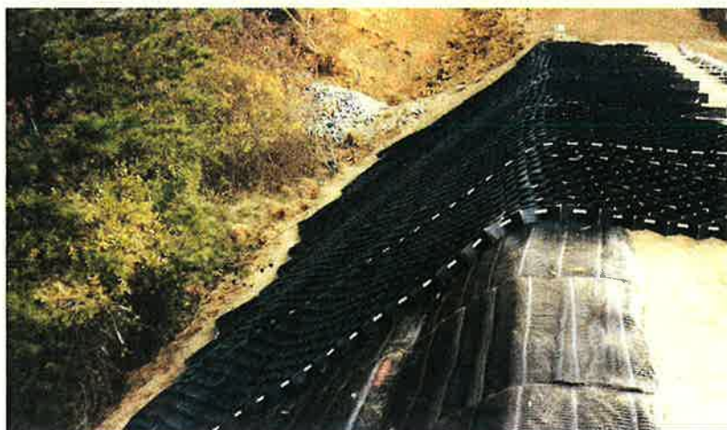
Photo 2. Cellular system anchored by tendons prior to fill.
