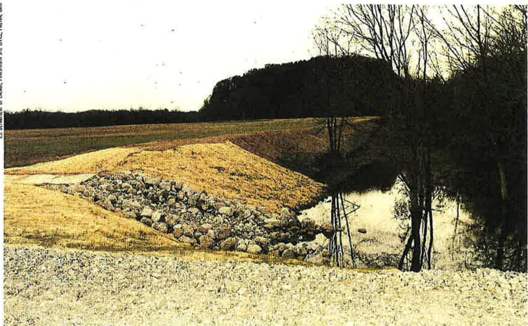
Photo 5. This photo was taken in late September 1996, after construction was completed.
