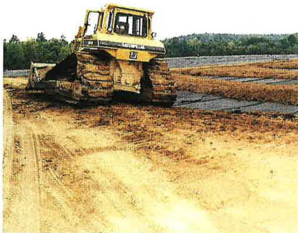
Photo 4. A large dozer placed soil over a previously placed soil lift. A smaller dozer was required to place the initial soil "fingers" and initial lift.
