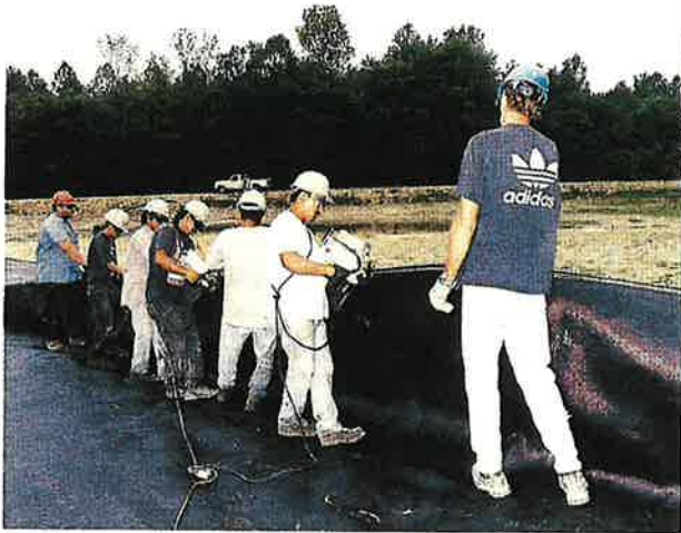
Photo 3. The field crews used a white thread to hand-sew the material so that it would be readily visible for inspection against the black geotextile.
