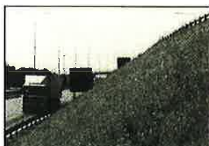
After: Same slope, lightly seeded, and later covered with a GREENFIX AMERICA blanket. The resulting vegetative cover was established in only four weeks.
