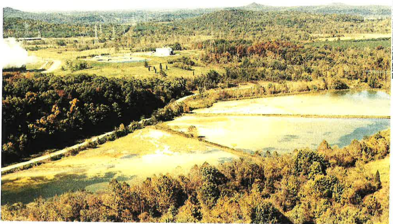
Photo 1. The sludge lagoons at the U.S. Department of Energy's Gaseous Diffusion Plant, before contractors removed nearly 85 million gallons of ponded surface water.
