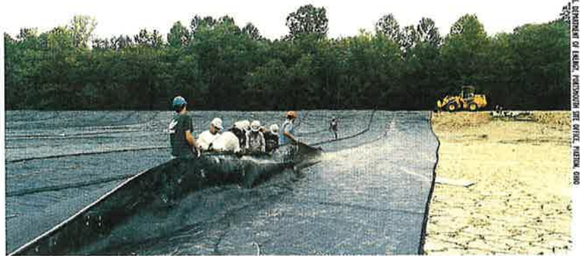
Photo 2. Contractors field-seamed the geotextiles as they placed the rolls.
