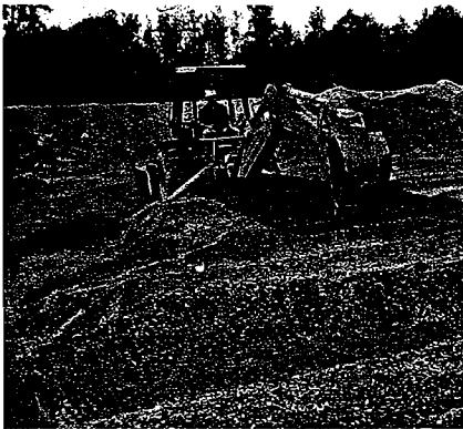
Photo 2. A small backhoe was used to carefully remove most of the stone with-out damaging the underlying geosynthetic.
