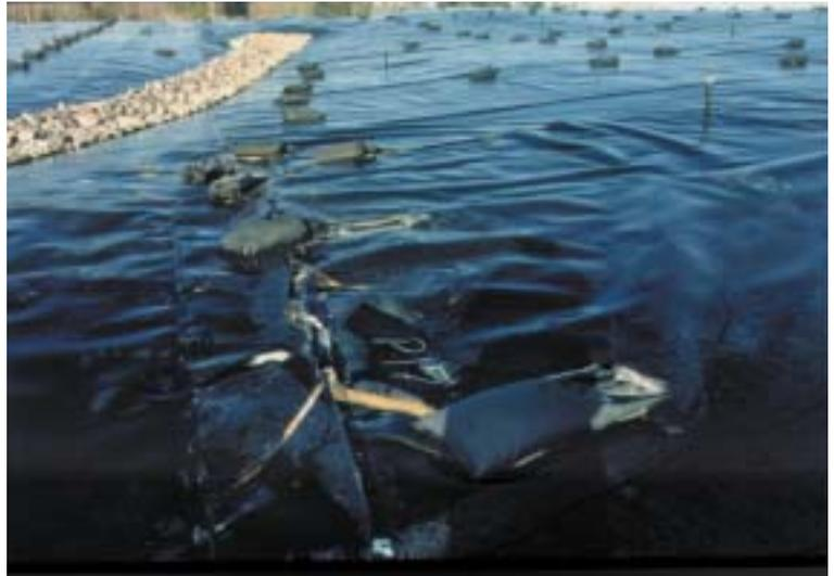
**Photo 1.** An interim closure using exposed geomembrane covers at the Department of Energy reservation in Oak Ridge, Tenn.
