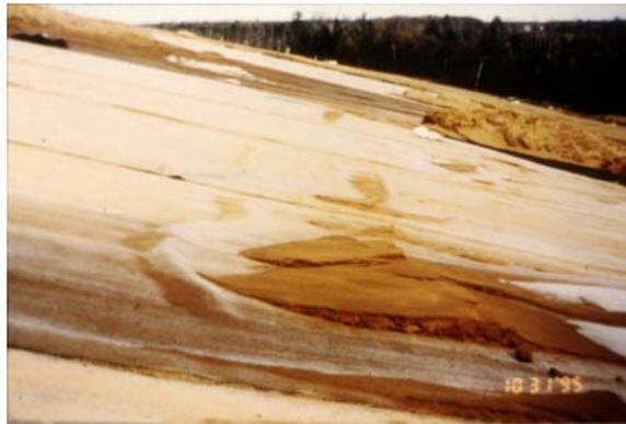
Figure 4 Sliding of Geomembrane and Sand Drainage Layer During Construction
