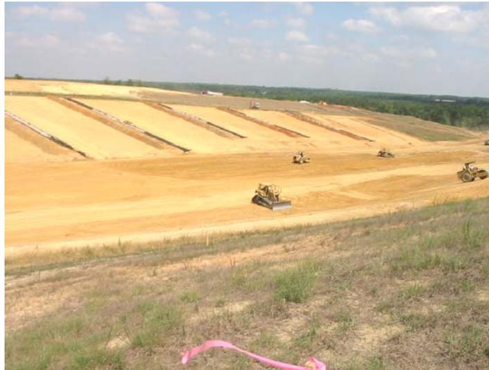
Figure 7 LFG Collector Trenches Installed in Surface of Existing Waste in Piggyback Landfill Application
