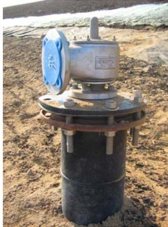
Figure 10 Emergency Gas Relief Vent
