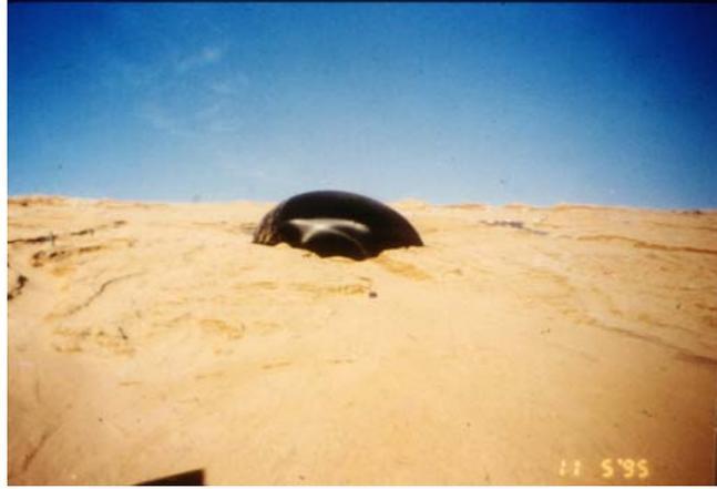
Figure 5 LFG 'Whale' Protruding Through Sand Drainage Layer
