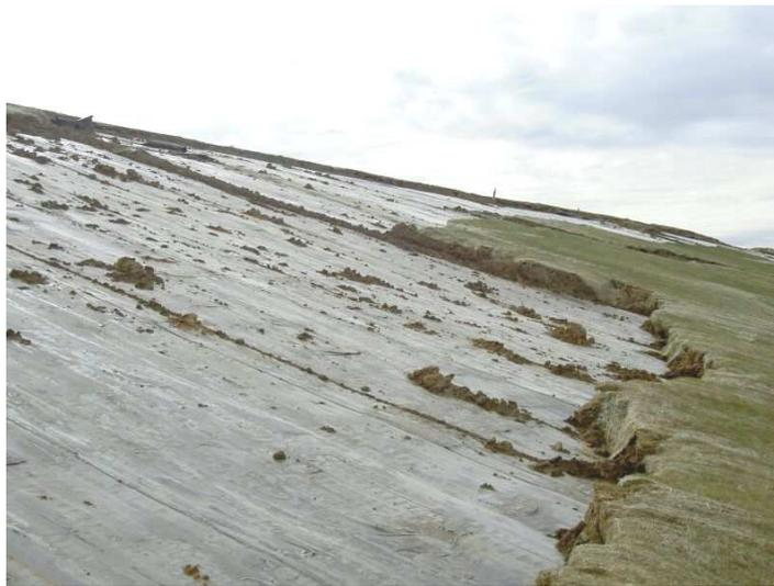
Figure 6 GCL Exposed by Final Cover Sliding Failure
