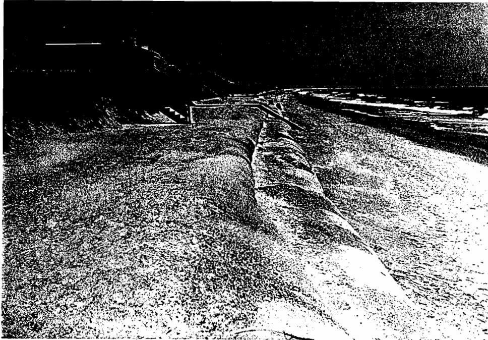
Figure 7 Completed Shoreline Erosion Control Tube System
