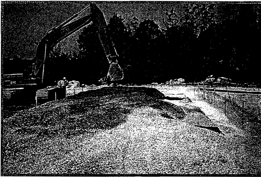
Figure 5. Placement of AASHTO #57 stone
