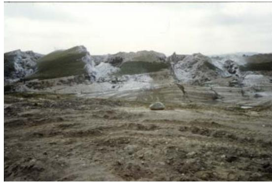
Figure 4 Landfill Waste Stability Failure
