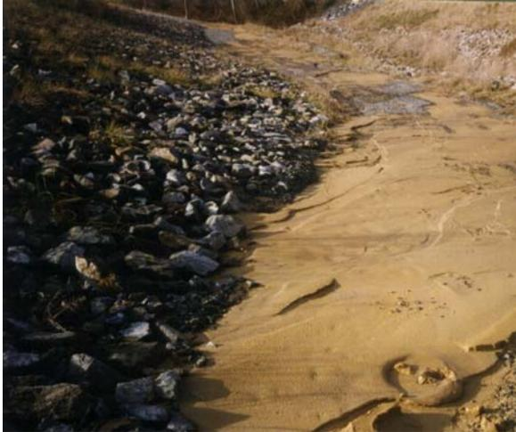
Figure 16. Vegetative support soils washed to slope base
