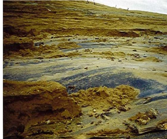
Figure 18. LFG buildup under the geomembrane
